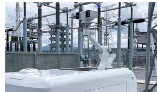
Power plant IR inspection
